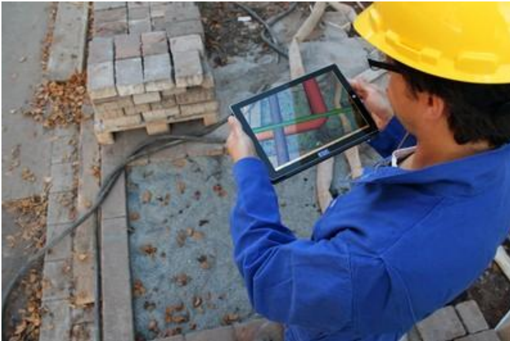
LARA: X-ray vision for civil engineering - augmented reality support for excavation work [Source: DFKI]
